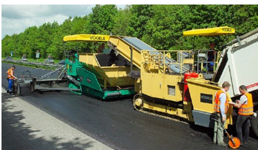
Figure 29 Road construction machines
